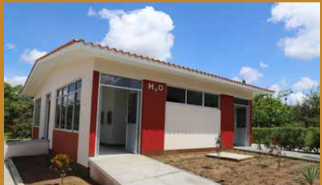
Partial view of H2O (Water Purification Plant). UNSIS. Miahuatlán de Porfirio Díaz
