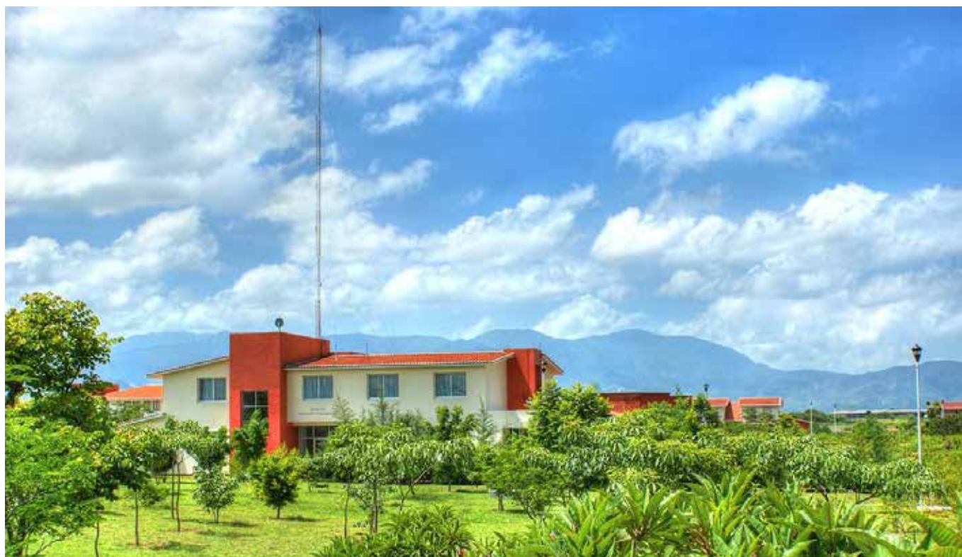
Transmission antenna. NovaUniversity. Ocotlán Central Campus.
