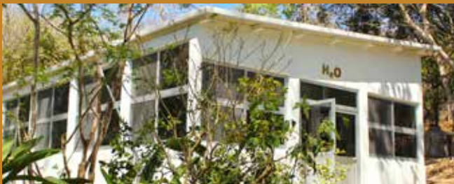
Partial view of H2O (Water Purification Plant). UMAR, Huatulco Campus
