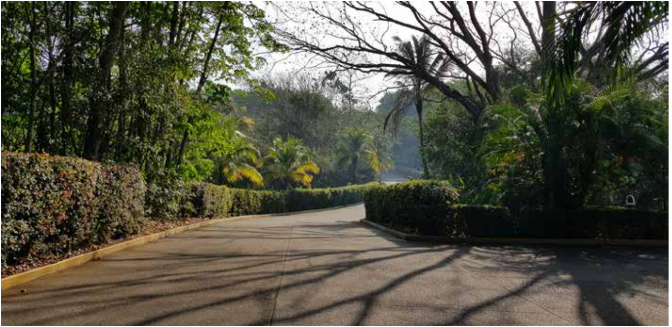
Vehicular and civilian access road. UTM. Huajuapán de León
