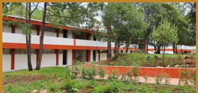
Classroom building and outbuildings. UNICHA. Chalcatongo de Hidalgo
